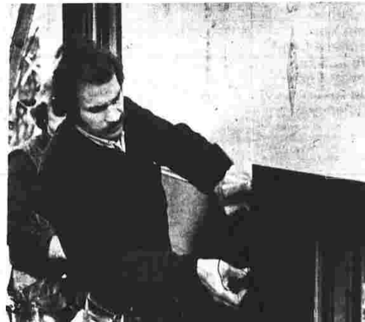
Styrofoam™ TG brand insulation can easily be incorporated into any standard residing job. The lightweight panels are nailed over the old exterior, providing a solid backing for the new siding. The new siding is then applied over the Styrofoam TG brand insulation, by nailing through siding and insulation into nailing substrate on original wall. Homeowners can reduce their home's energy consumption and realize annual savings in their heating/cooling bills by adding this board-form sheathing product to their home's exterior sidewalls. Styrofoam TG brand insulation can pay for itself in energy savings within approximately four to five years time. *Trademark of The Dow Chemical Company
